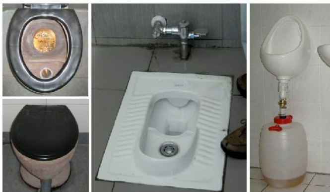
Fig. 1: Selection of sanitary installations for urine collection. Flush-less sitting toilet (Ghana), squatting pan (China) and home urinal (Germany)
