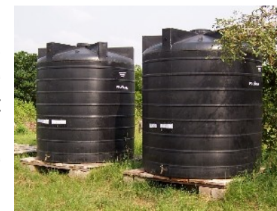
Fig. 2: Urine storage tanks close to agricultural fields (Ghana)
